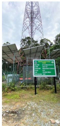
Deployment of solar-powered gensets at remote sites
